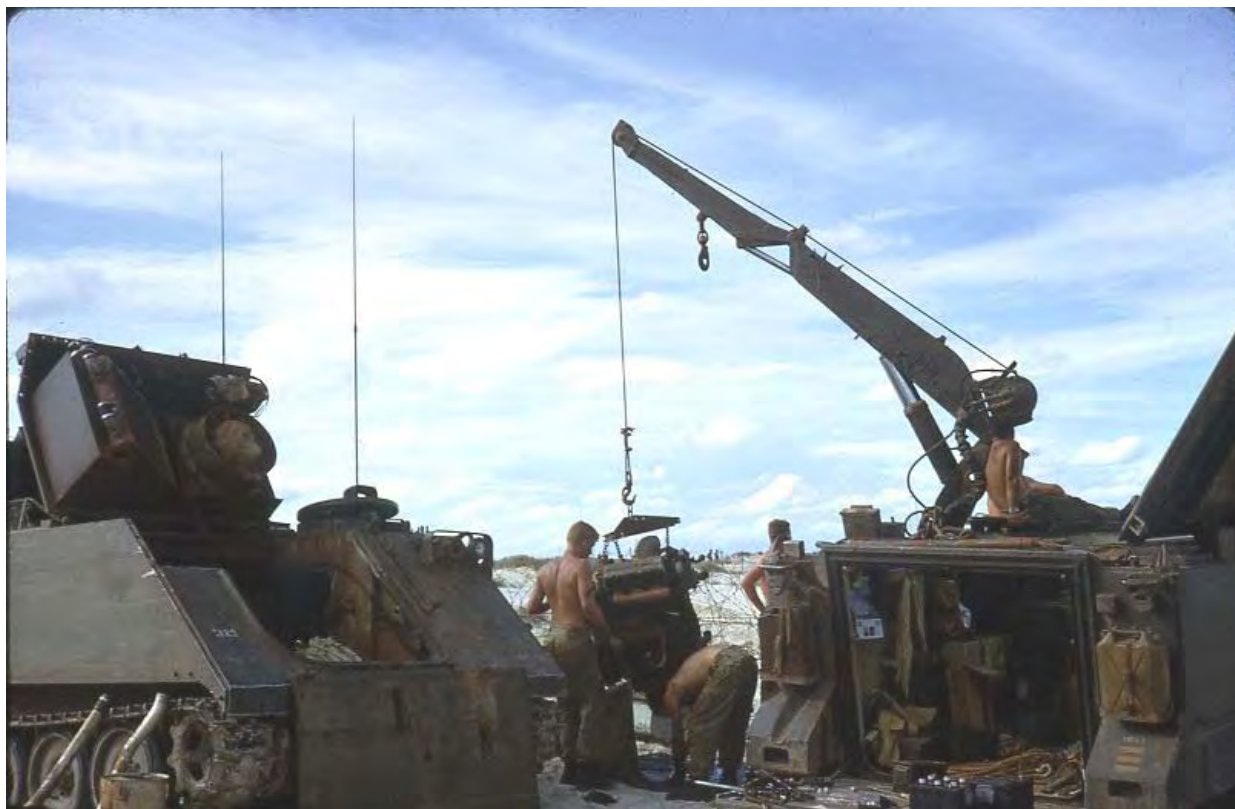
A SQN 3 CAV LAD changing an M113 APC engine on Operation Leeton May 1967
